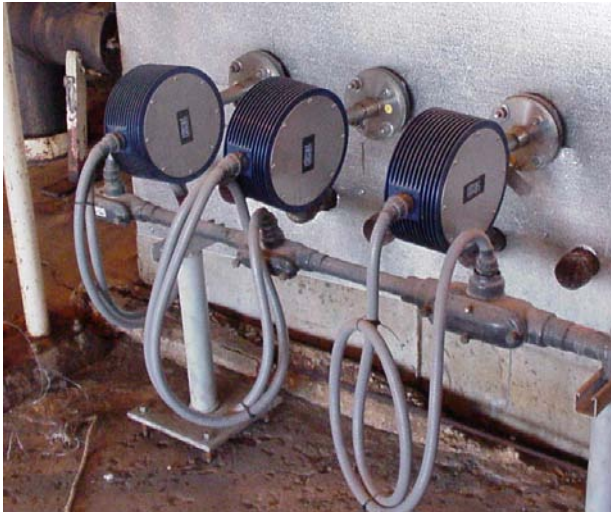
Figure AH-5. Flex sensor connection for service loop, TA version using Liquid Tight Conduit.
